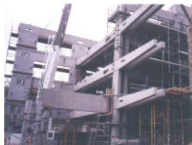
The 300mm thickness of all sections created extreme congestion of reinforcement and continuity ducts particularly at the cantilever support points where elements interacted in three directions.
