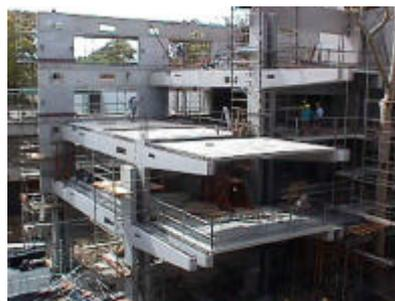
The structural design and buildability for transfer of the tension force from the cantilever and inclined strut to the anchor block was the unusual design feature of the project. A number of options were considered. These included:
