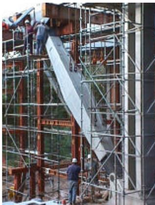
Application of this technology combined with a rigorous manufacturing procedure allowed a superior, high class F1 off-form finish to be achieved on all elements.
