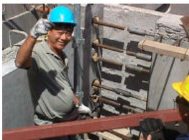
After extensive consultation with the specialist precast concrete designer/supplier, the CADWELD system was adopted for mechanical coupling of the main tensile reinforcement. While this system has been used extensively in overseas projects, this was the first use of this coupling system in an Australian building. The unique advantage for its choice was the compactness of each joint, resulting in a hidden in-situ pour strip only 600mm long at each joint.
