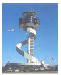
The control room complex is supported on a 20m high segmental precast shaft, 2.5m in diameter but with a truncated flat face against which the passenger lift structure is fixed. This shaft is also vertically stressed, but in stages to its foundation using 31 No high strength post-tensioned bars which connect directly at the top of the shaft to the upper steel control room support column, thus providing its stability.
