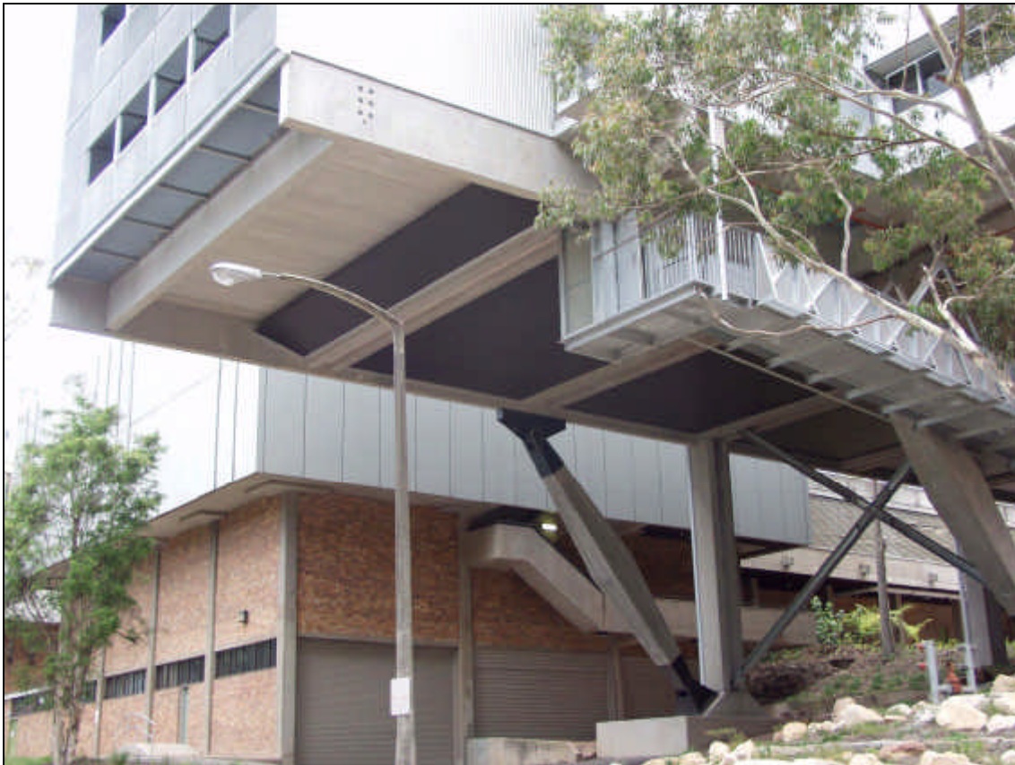
Display of Huge Cantilever and Concrete Tension Ties
