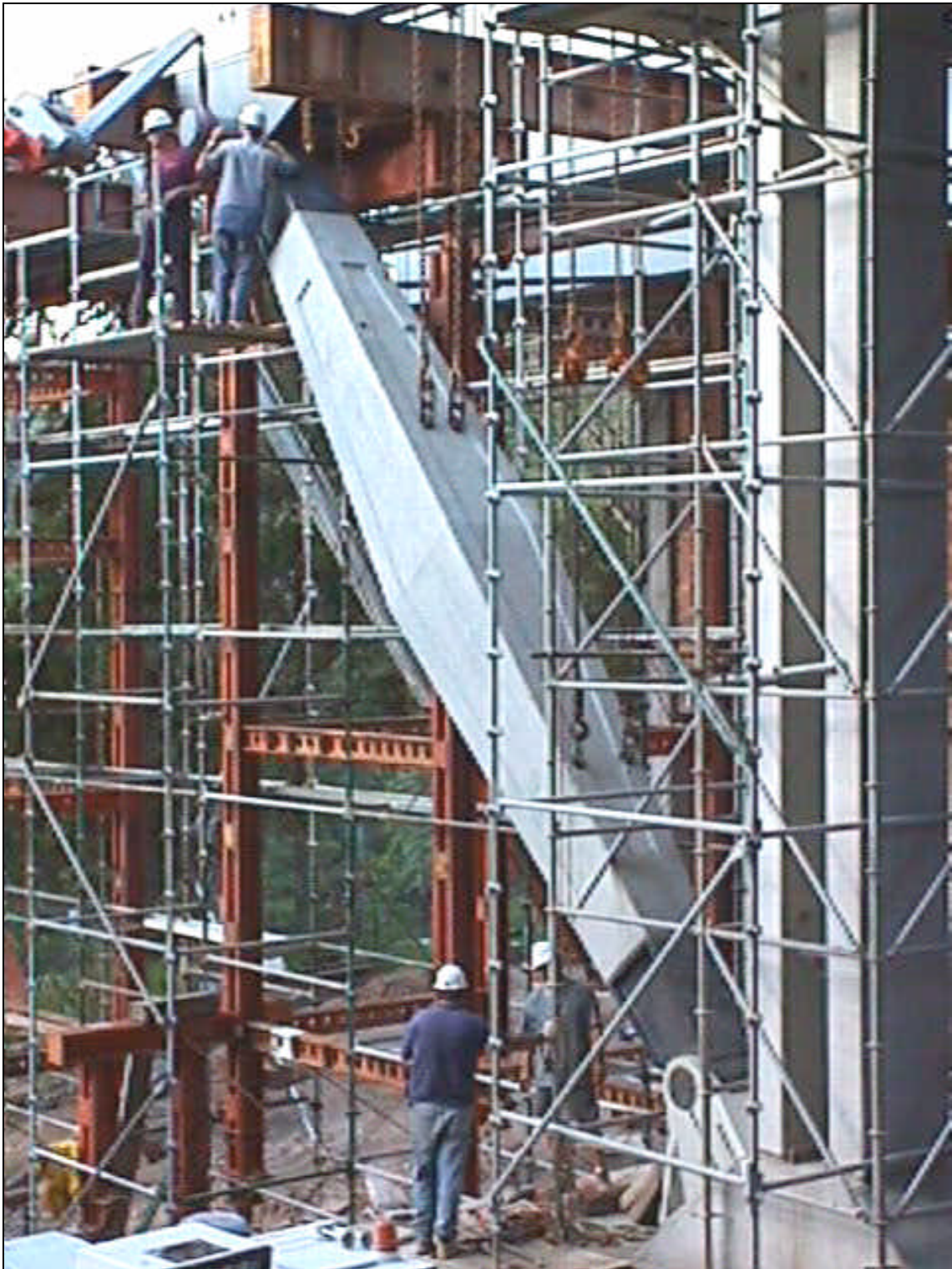
Erection of strut
