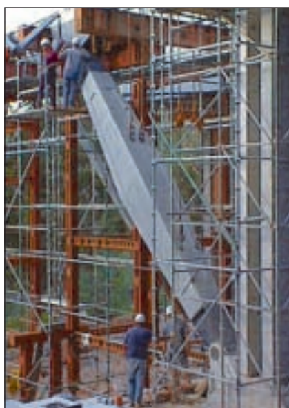
Erection of precast spandrel tension tie (note temporary stability support for wall)
